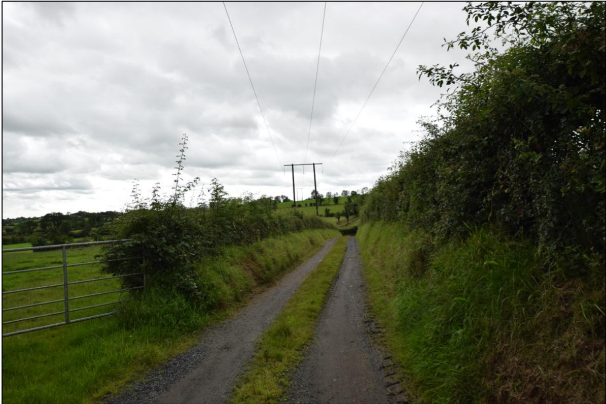
Plate 1: Existing Lisdrum-Shankill 110kV electricity transmission line to which the proposed development will connect.
