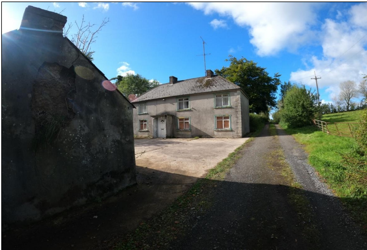
Plate 4: Residential and farm buildings are located in the vicinity of the proposed development site.
