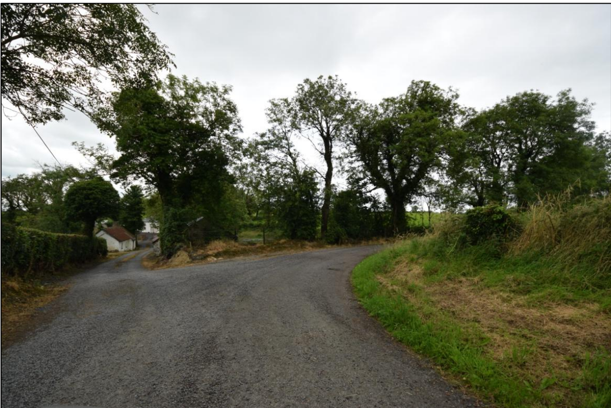
Plate 2: Location where proposed underground electricity line will be located adjacent to LT62013
